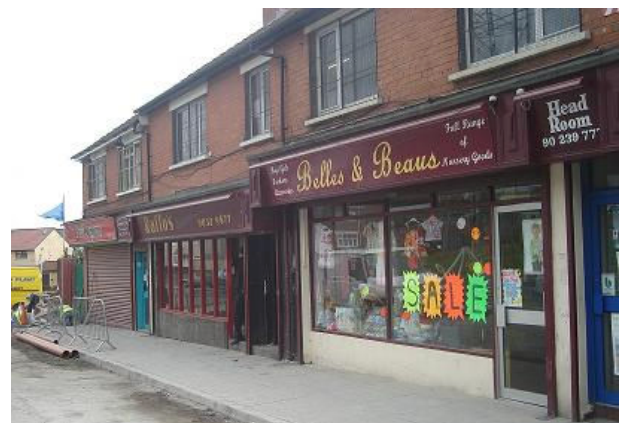
Springfield Junction project during construction
